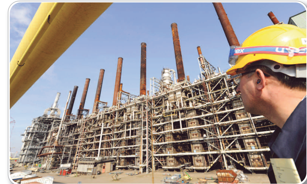
The configuration and performance of Moerdijk's ethylene cracker, a large contributor to CO2 emissions due to the high operating temperatures involved, came under close scrutiny as part of the study.
