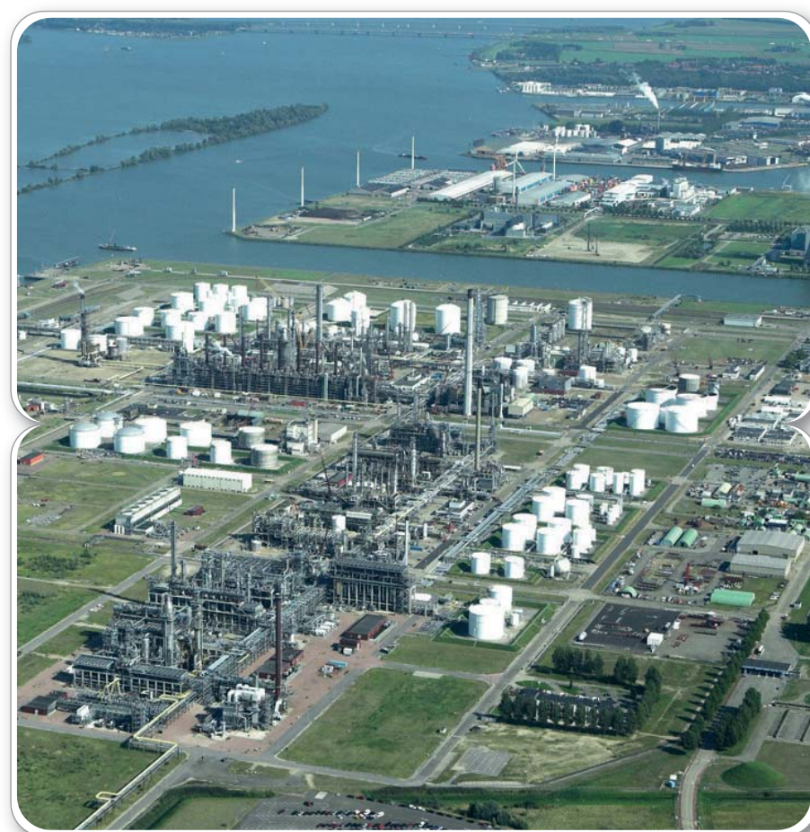
The Moerdijk plant in the Netherlands has been used to develop a framework for a range of realistic and measurable energy efficiency and carbon abatement measures to reduce emissions.
