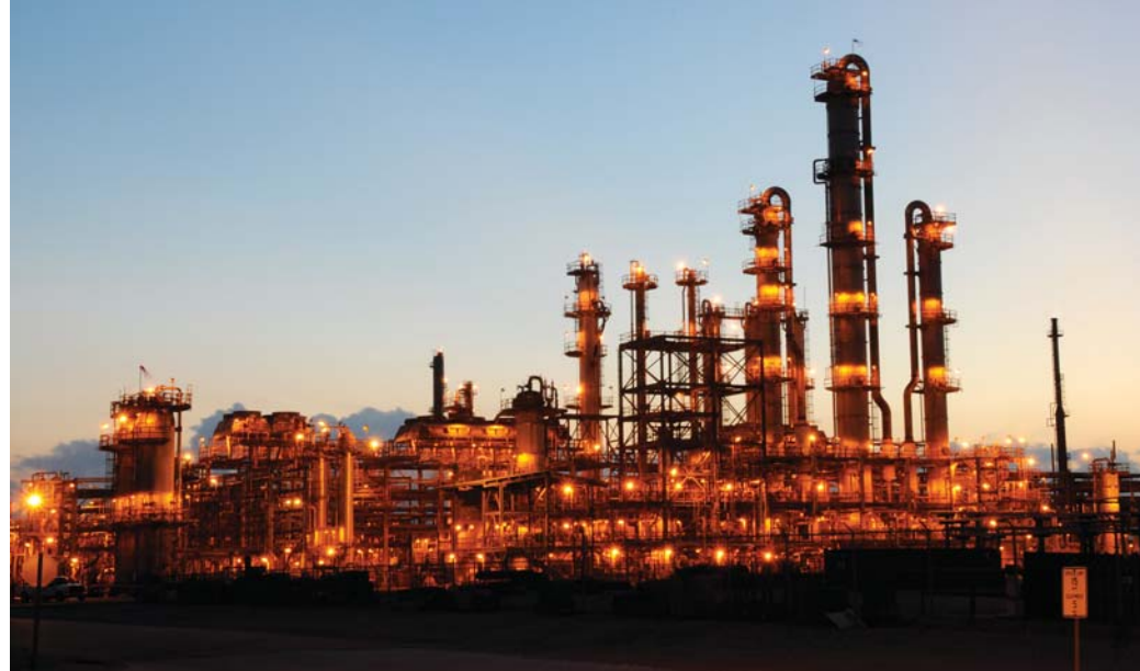
Shell's Geismar, Louisiana, alcohols production complex is the largest in the world and has the capacity to process additional volume of oleo alcohols.
