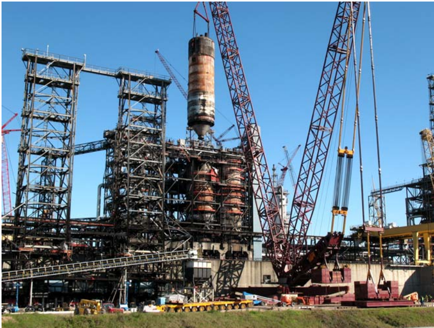
COKE DRUM REMOVAL
