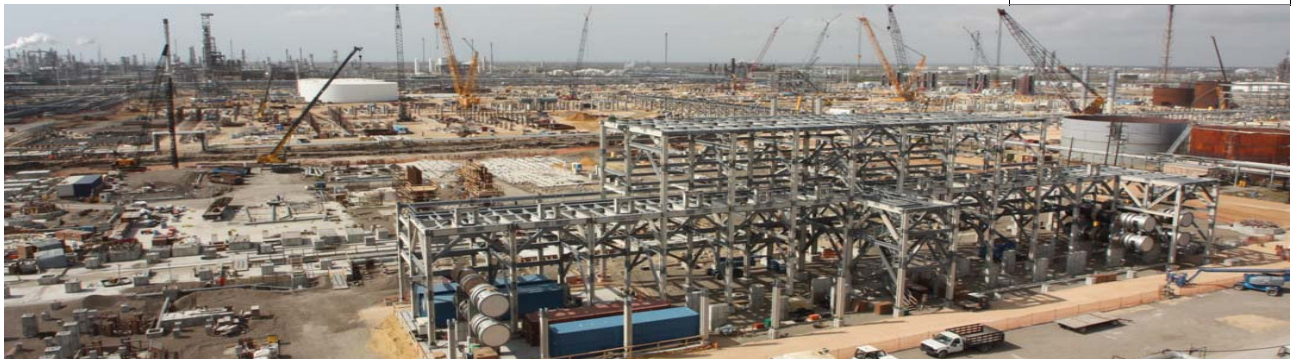
Figure 1: Motiva refinery expansion, Port Arthur, USA
