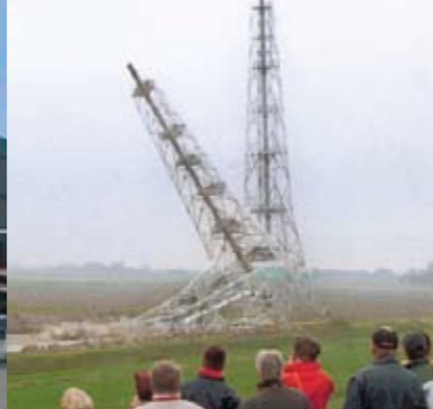
Characteristic flare stack is demolished
