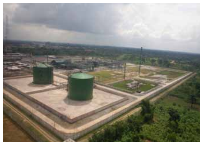
Okoloma gas plant
