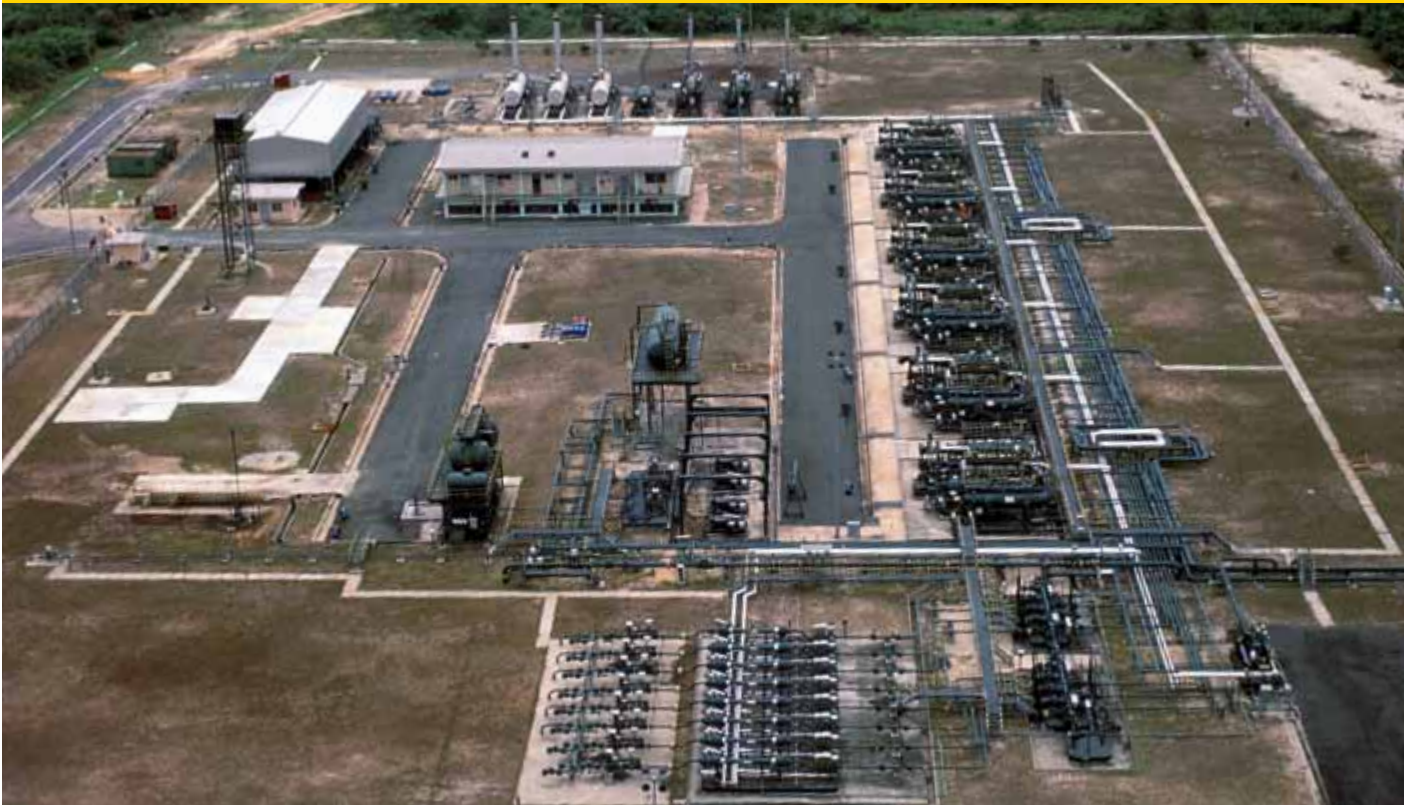
Aerial view of SPDC's Utorogu gas plant
